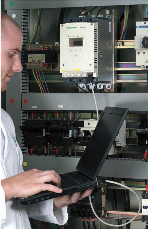
Testing and start-up of the ATS 22 soft start/soft stop unit using SoMove setup software
